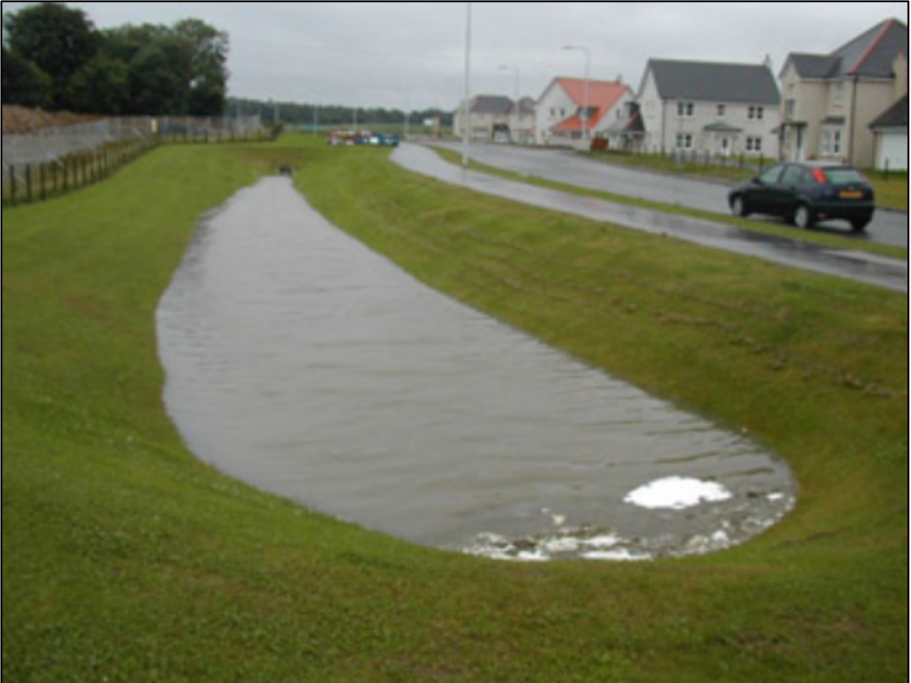
Figure 4: Typical Detention Basin
